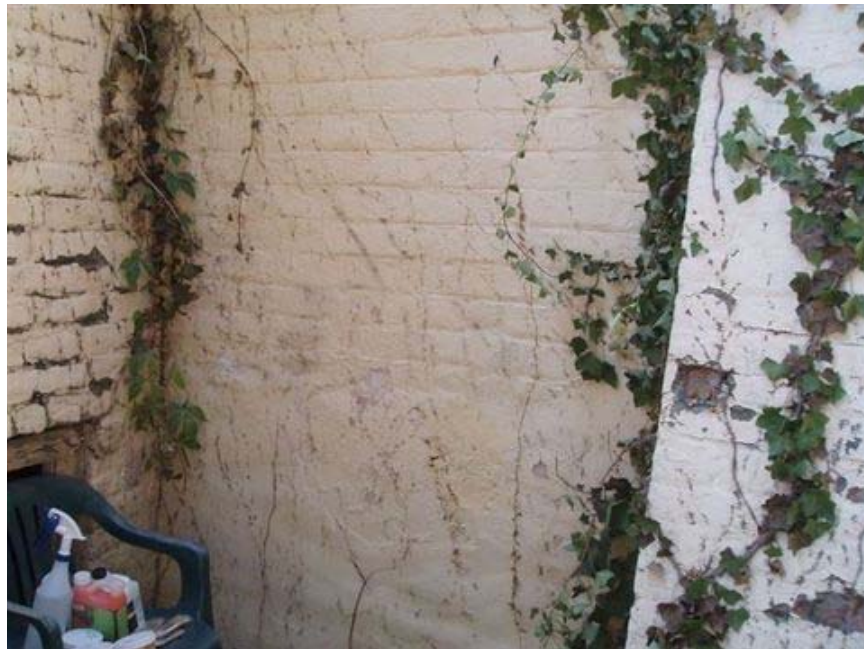
Figure 1: During Testing, Exterior Masonry Wall Prior To Test
